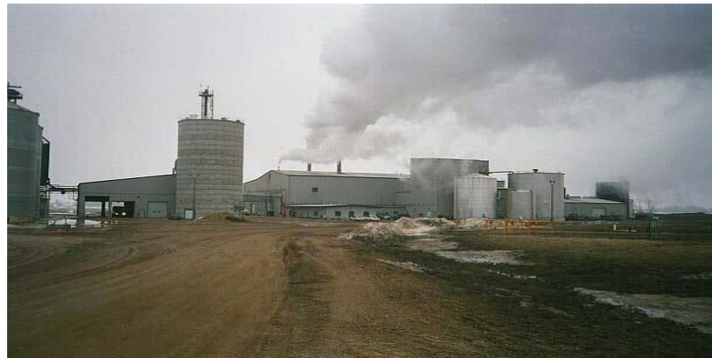
SMAC plant, Bingham Lake, MN
